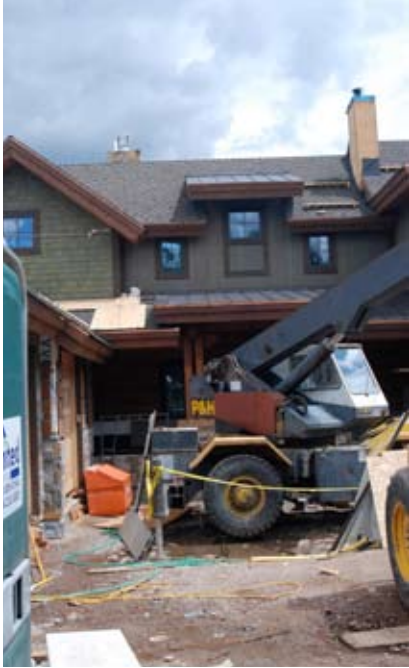
A new home being constructed in the Cemetery Lane neighborhood.
