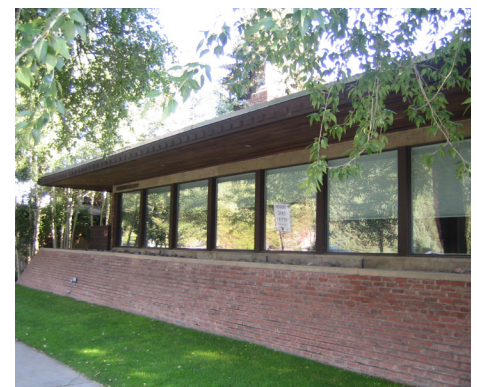
The old library building, located on Main Street across from Paepcke Park was designed by Fritz Benedict, and is an example of Aspen's Modern Architecture.
